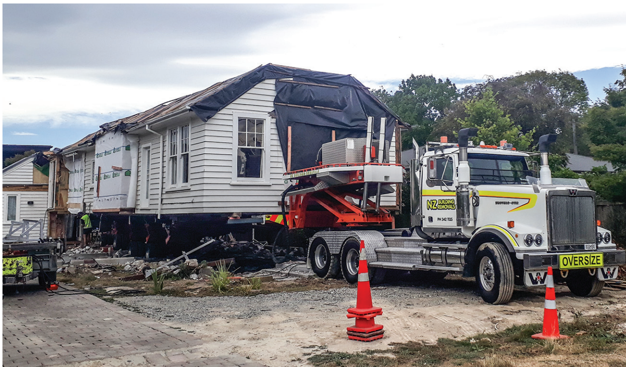
Figure 23: Timber framed residential building in Christchurch being relocated for reuse (K. Symons).
