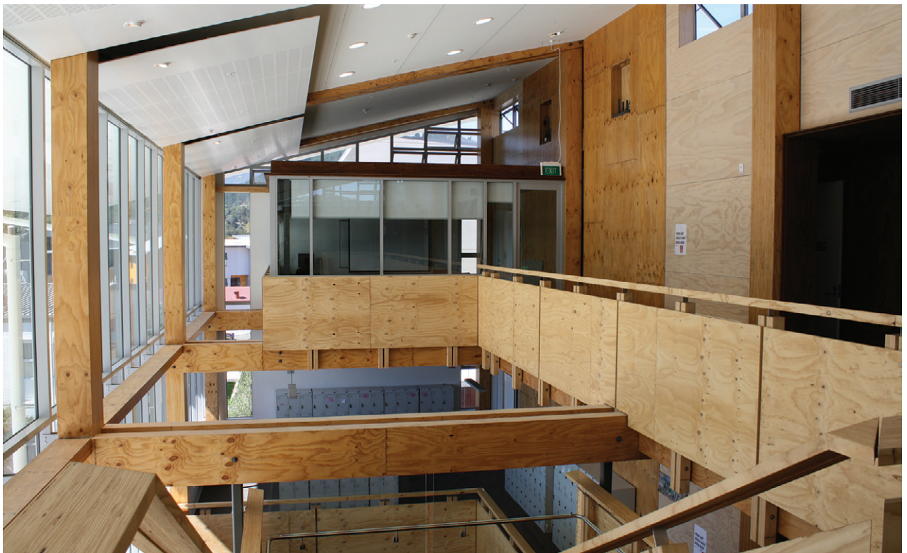
Figure 30: The NMIT building made use of an innovative post-tensioned timber frame, with seismic resilient technology .
