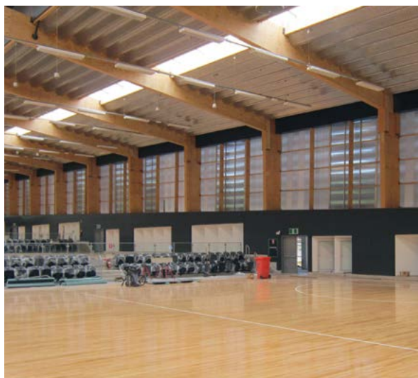
(Above and below) NSW Netball Center using LVL portals and Quick Connect Connections
