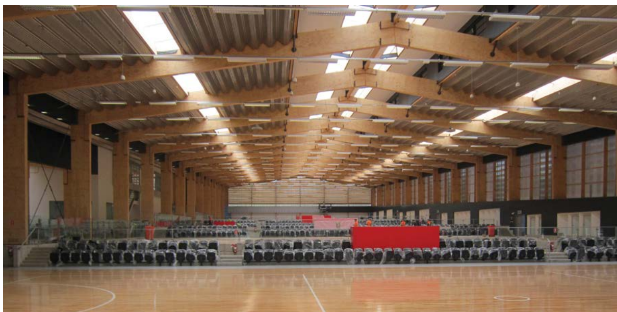
(Above and below) NSW Netball Center using LVL portals and Quick Connect Connections
