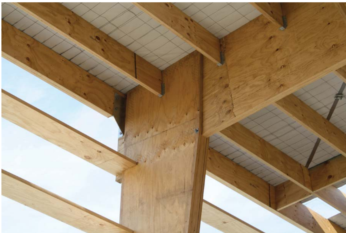
Figure 6 Lap Joint
