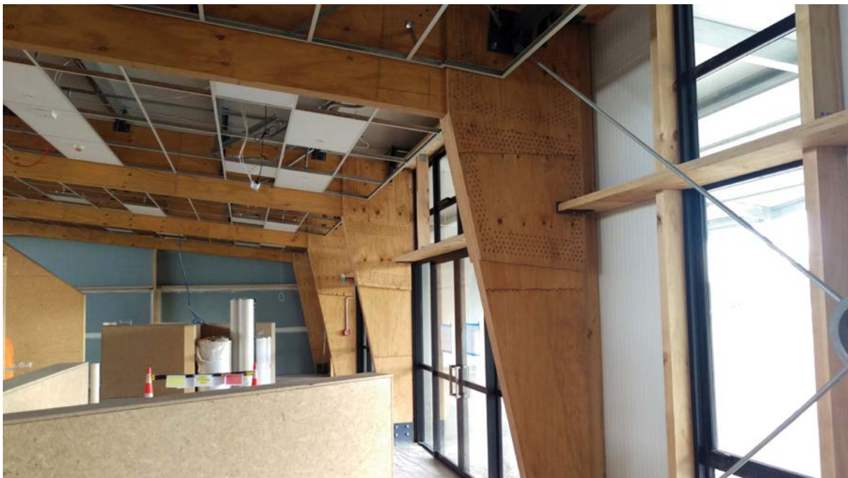
Marshlands School using LVL portals and LVL gussets.
