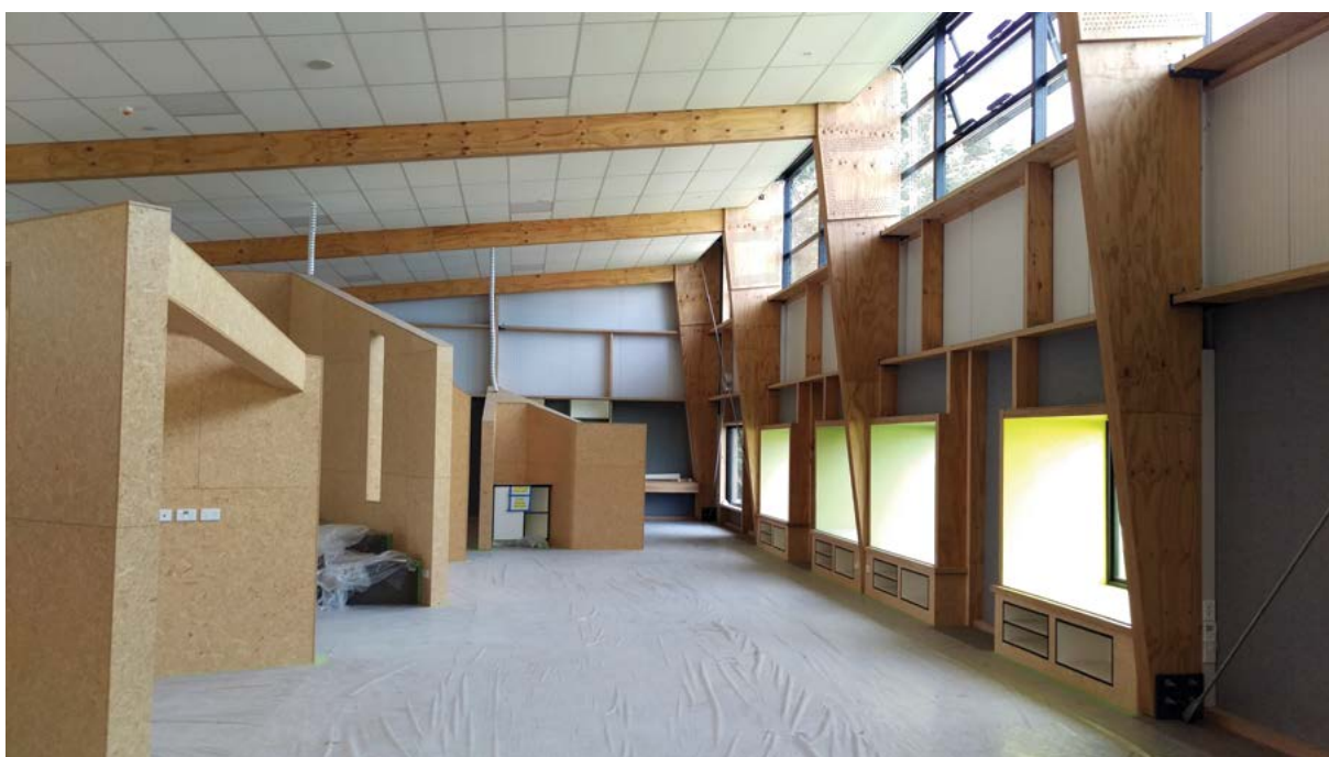
(Above and below) Marshlands School using LVL portals and LVL gussets.
