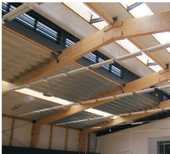
(Above and below) NSW Netball Center using LVL portals and Quick Connect Connections
