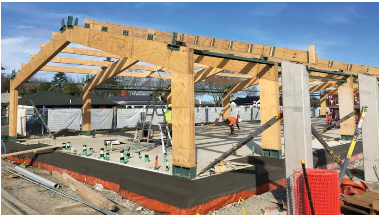
North Canterbury Schools, using LVL portals and WS dowels and steel plates
