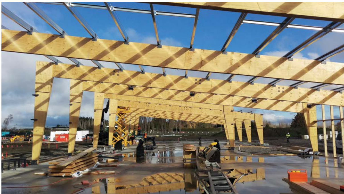
(Above and below) Marshlands School using LVL portals and LVL gussets.
