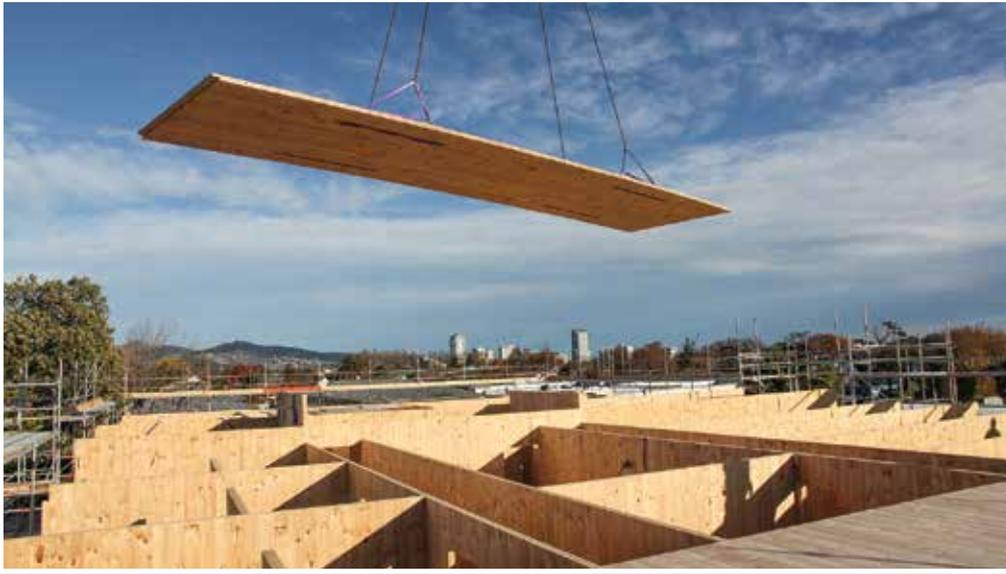
Honeycomb structures are well suited for CLT panel construction. (Photo: Xlam NZ Ltd).
