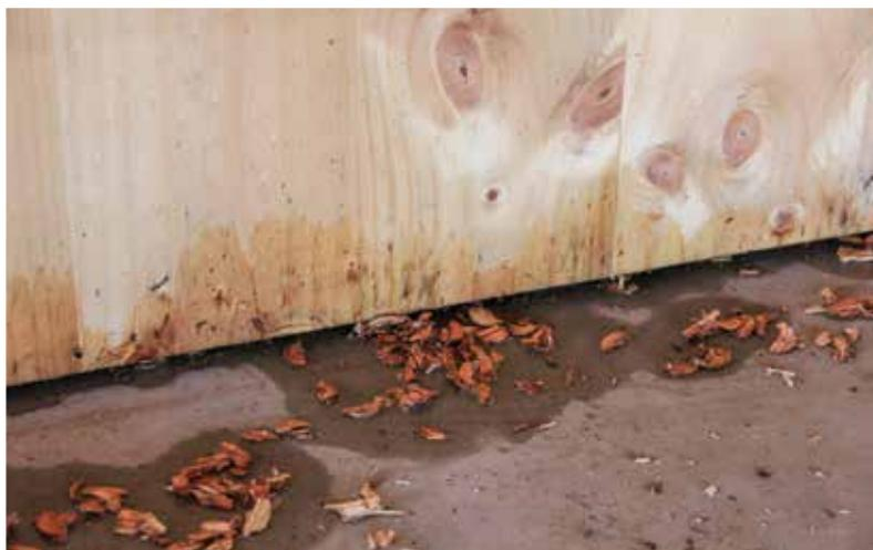
*Unprotected end grain taking up ponding water.
