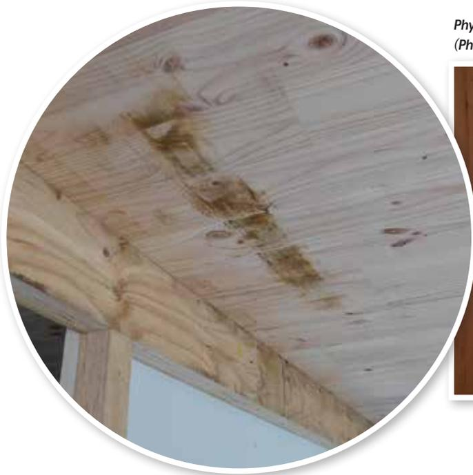
*Marked surface due to forklift prongs. (Photo: Xlam NZ Ltd).*
